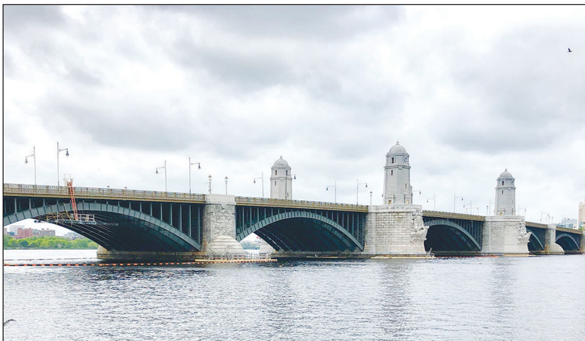
The Longfellow Bridge.
