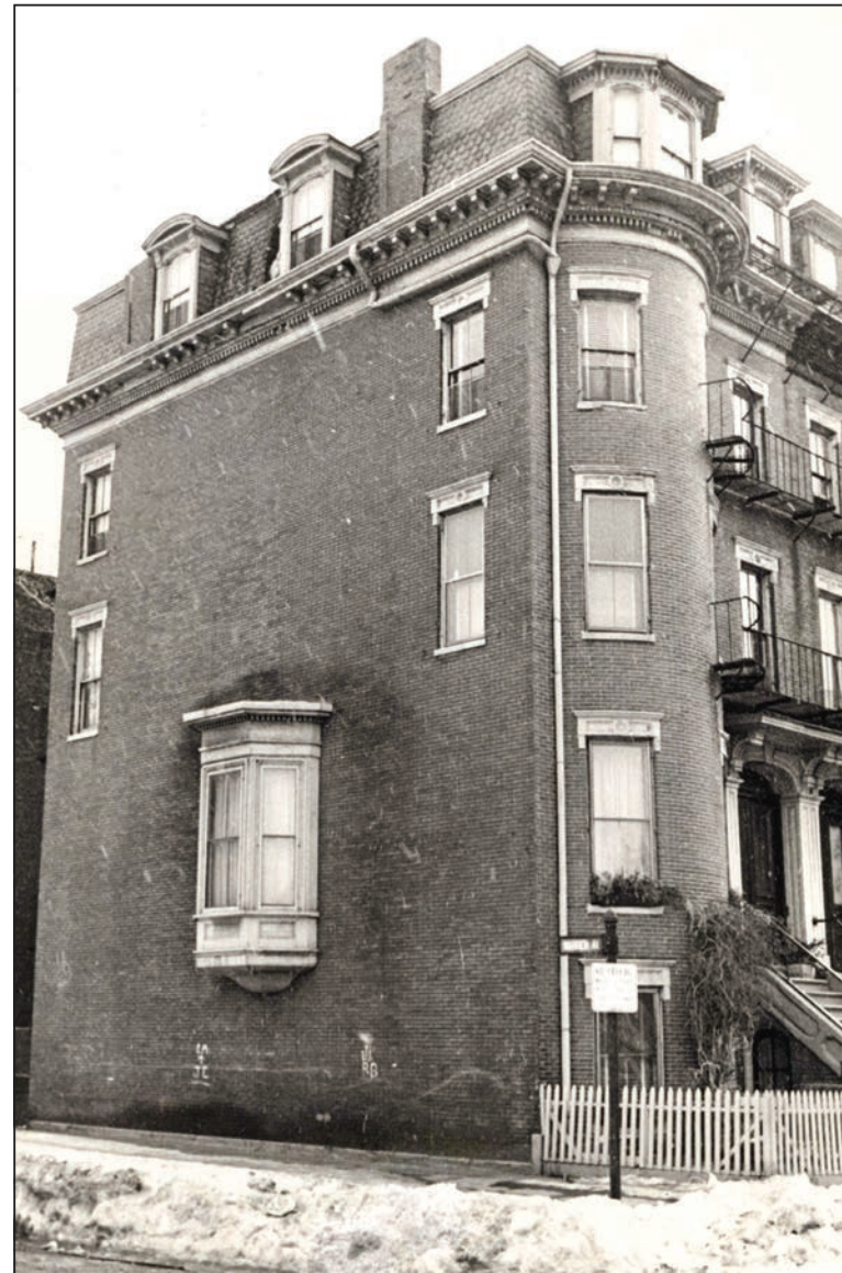
The oriel window in the last clue is on the Warren Avenue side of 141 Pembroke Street, built circa 1900. Today's answer is a Boston Redevelopment photo from the 1970s. It shows how a detail like that can change over time without the protection of The South End Landmarks District.
