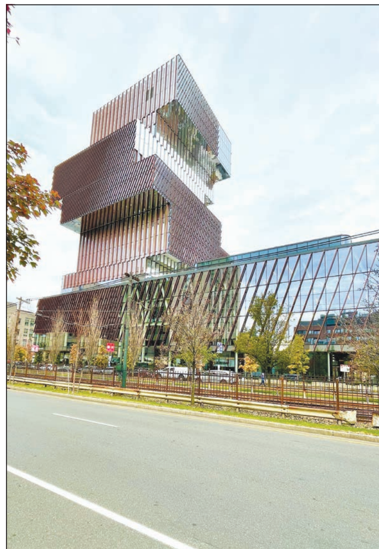
The striped section in the last clue is on 665 Commonwealth Avenue, BU's Center for Computing & Data Sciences. The design features multiple cantilevers, which are more of an engineering feat than an architectural one. The Forth Bridge in Scotland, built in 1890, is one of the earliest examples of this engineering technique and is still used today.
