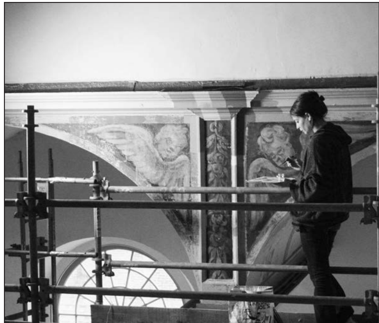
A restorationist works on the angels.
