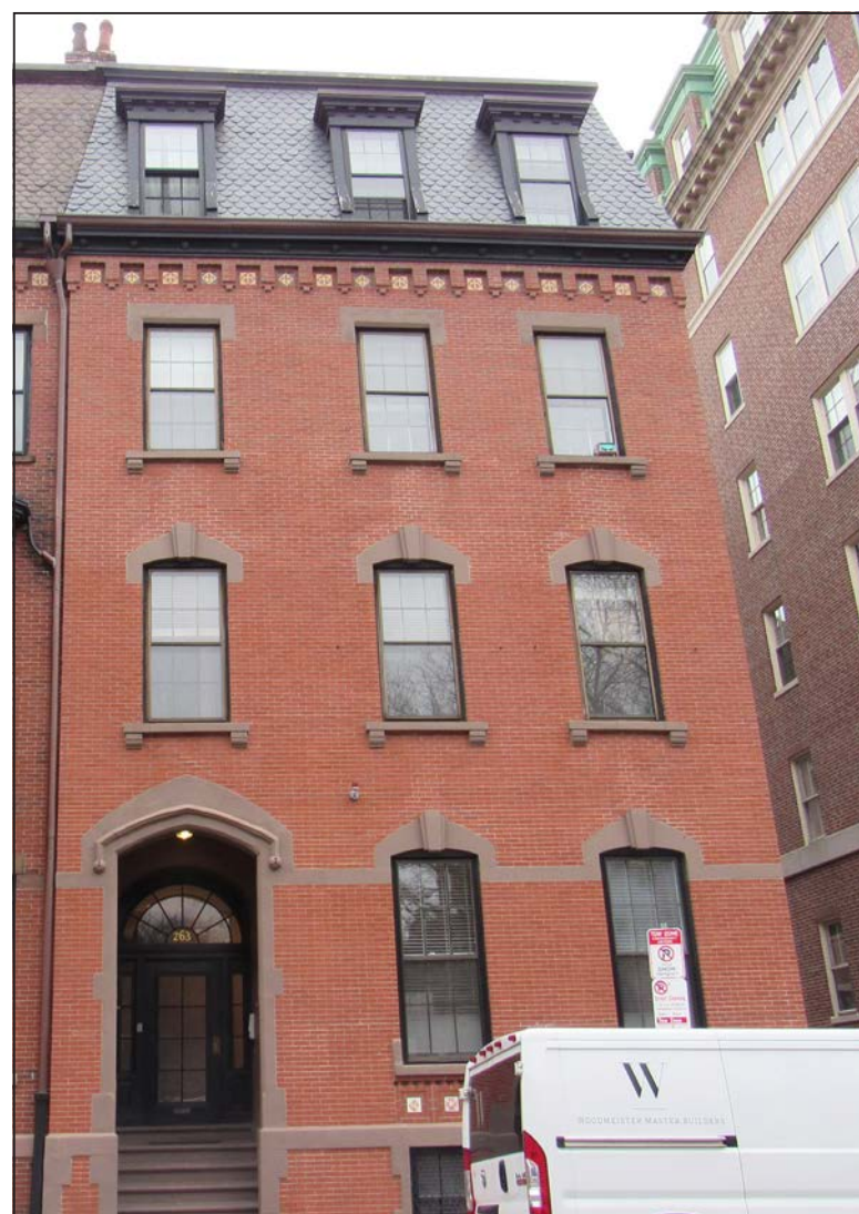
A property at 263 Clarendon St., which The Learning Project intends to transform into additional classroom and administrative space.
