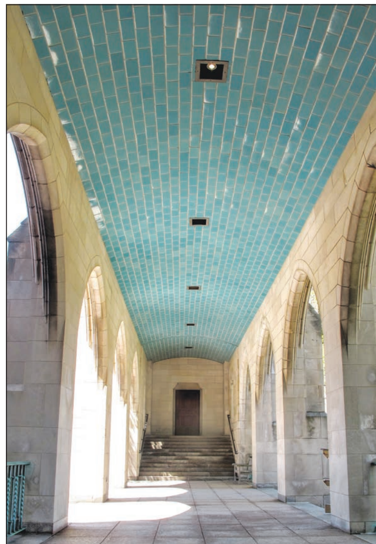
The last clue's tile detail is on the cloister walkway at BU's Marsh Chapel. This is a publicly accessible example of the Guastavino tile arch. Architect Rafael Guastavino patented this structurally strong and fireproof system in 1842, and it was used in many Boston buildings, including the Boston Public Library in Copley Square.
