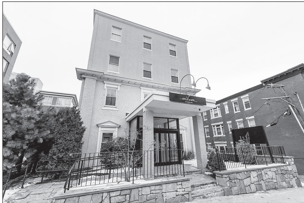
The enVision Hotel at 81 South Huntington Avenue.
