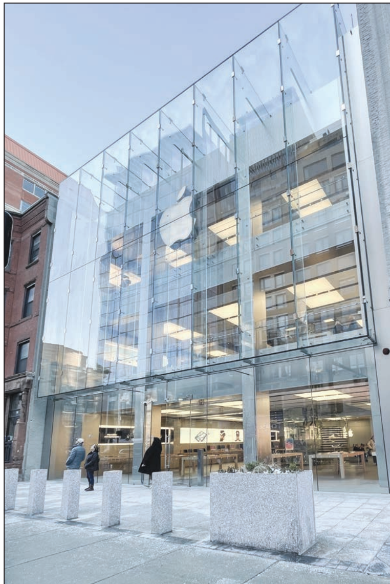
The window array in the last clue is on the Apple Building at 815 Boylston Street. It was opened in 2008, and in January of this year, Apple purchased the property from Tribeca Holdings for 88 million dollars.
