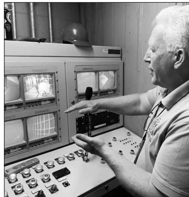
The new SCBA Maze Trailer replaces a 40-year-old permanent installation with obsolete electronics, seen here, that has exceeded its useful lifespan.
