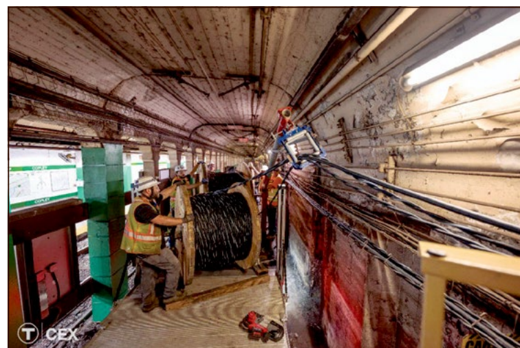
Workers running new cable inside of Copley Station.
